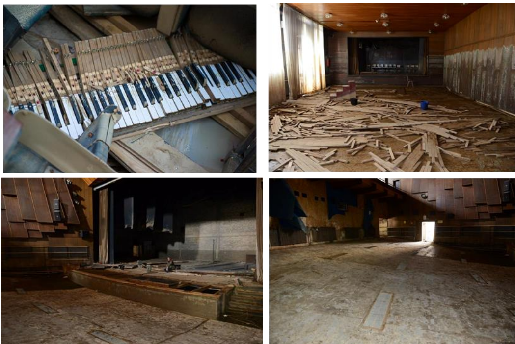
Figure 1-38. Cultural center of Obrenovac. The situation after the withdrawal of water. The picture top right shows the small theater hall, the line of flooded level is evident. The two pictures bottom right and left show the great theater hall after the remove of parterre seats and the damages to the revolving rotation system of the theatre stage. theatre hall. It will take around 6 months for the recovery of the theatre. The loss income is estimated around EUR 2000 per month.
